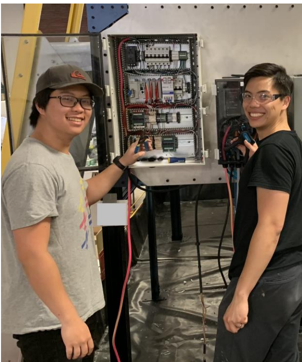
Figure 1: Pilot Plant under construction at Lilac's facility in Oakland, California. Lilac materials engineer Garrett Lau (Ph.D. Northwestern University, B.S. Massachusetts Institute of Technology) and process engineer Amos Indranada (B.S. University of California Berkeley) showing the controls.
