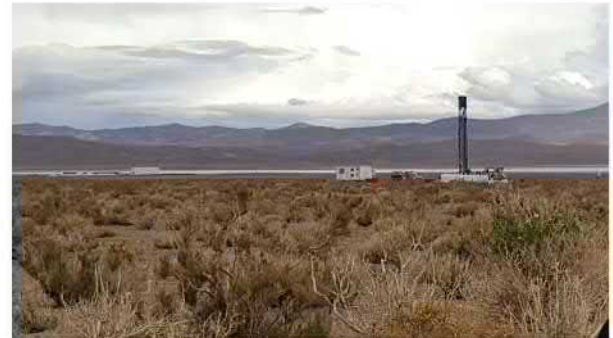
Cauchari West I nearby Advantage drill rig and Lithium America camp
