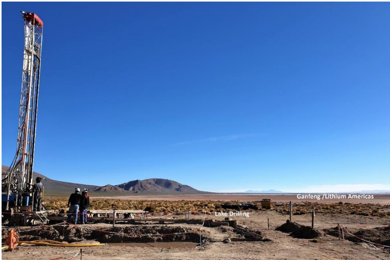
Figure 3: Rotary rig currently operating at site and at 234m deep
