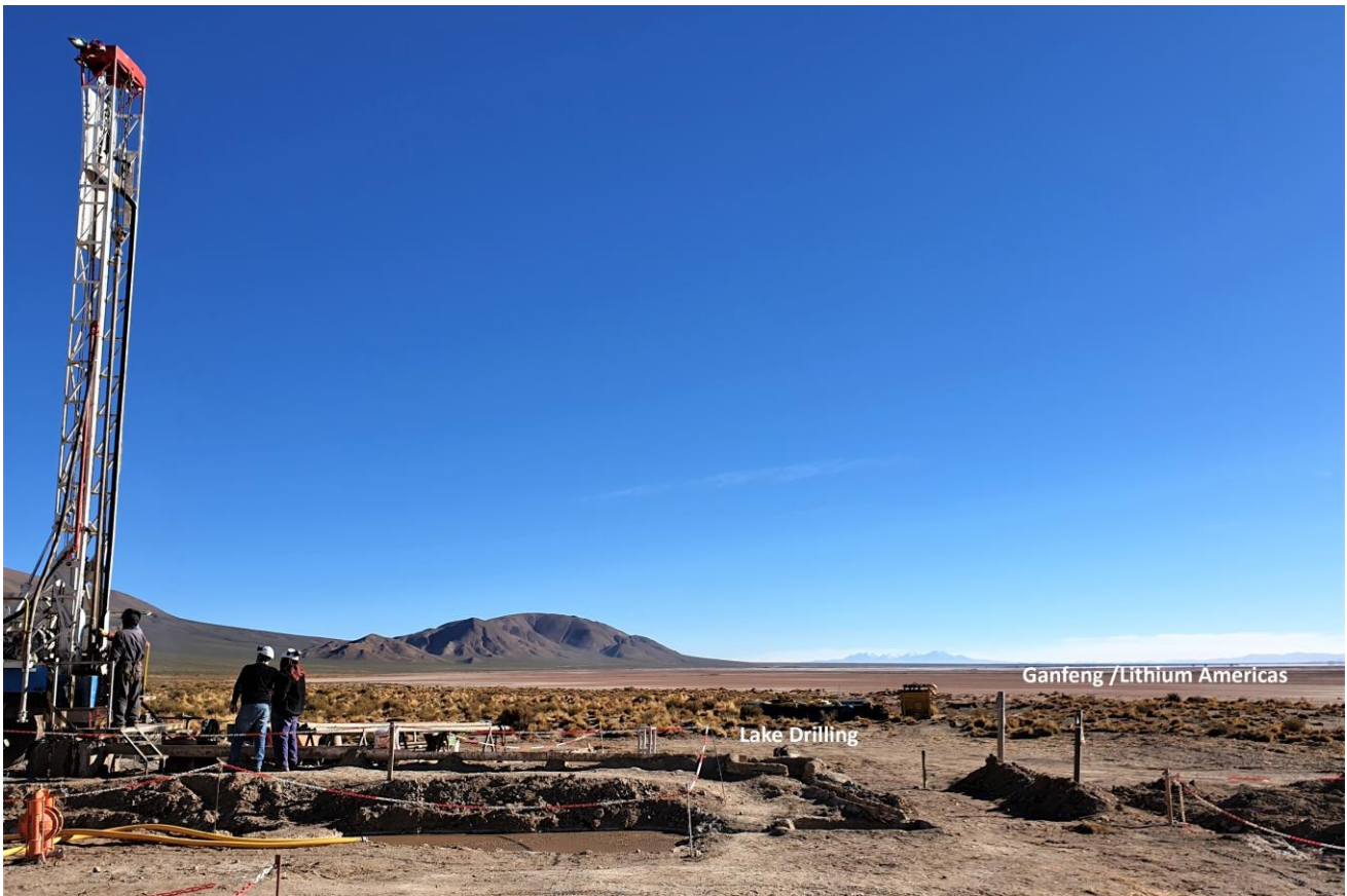
Figures 3: Rotary rig currently operating at site and at 234m deep
