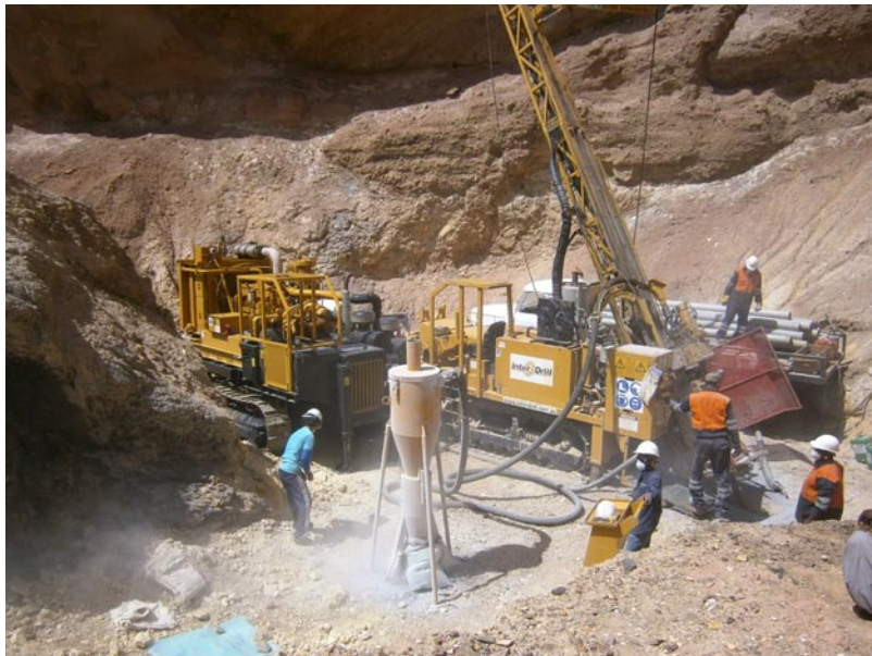
Figure 4: Drill Site LRMRC-003 Crawler-mounted compressor on left, multi-purpose drill centre and cyclone sample collector front-centre.
